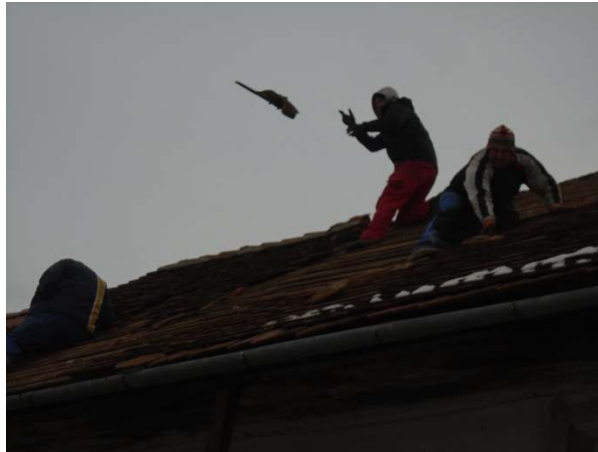
Action shot of the tiles flying off the roof!
